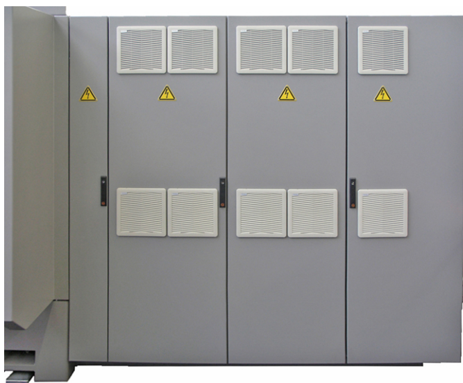
Example: Filter on the control cabinet
